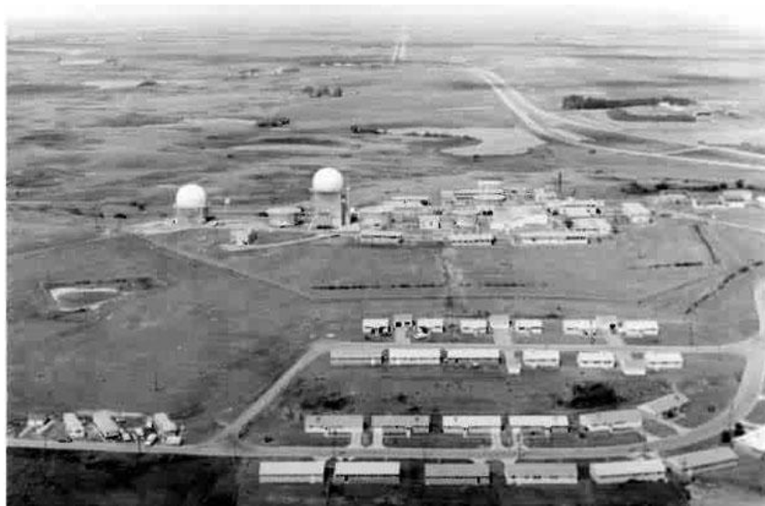
Minot Air Force Station, ND, looking north. The radar systems consisted of a Westinghouse AN/FPS-26A Frequency Diverse height-finder and AN/FPS-27 FD search radar, designed to have a maximum range of 220 nautical miles and search to an altitude of 150,000 feet. Regarding the AN/FPS 27 FD system, and Minot AFS
